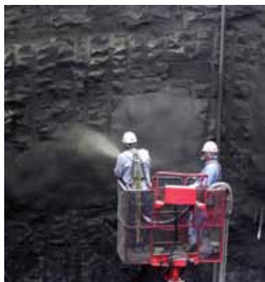
QUIKRETE Shotcrete MS used in a mining application
