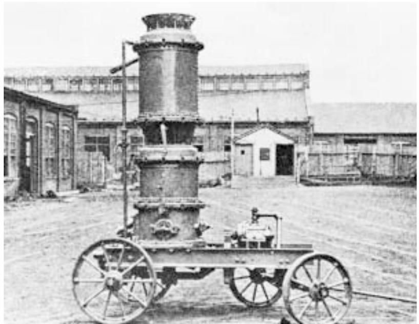
*The original machine used in 1907 to recoat the facade of the Field Museum of Chicago.*
