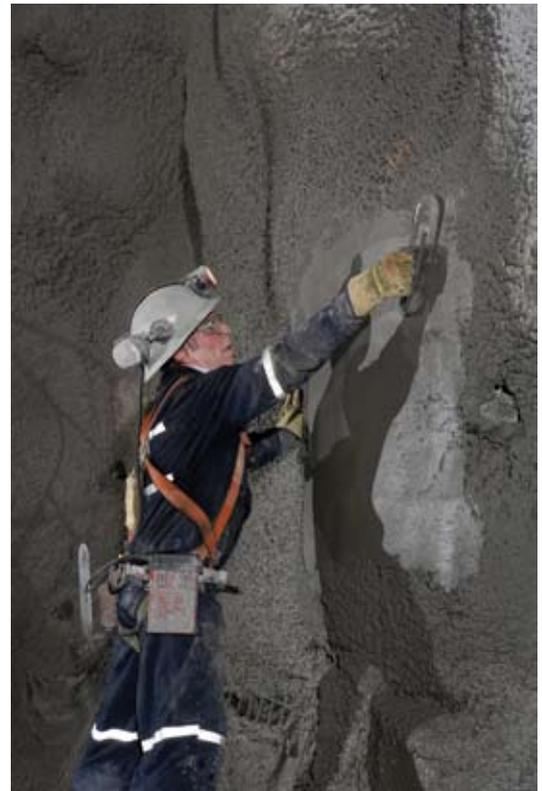
Fig. 4: Trowelling of finish shotcrete layer
