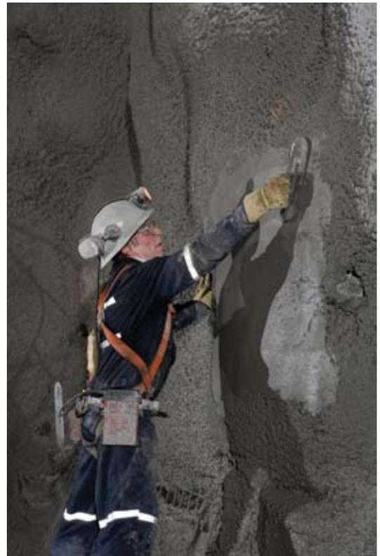
Fig. 4: Trowelling of finish shotcrete layer
