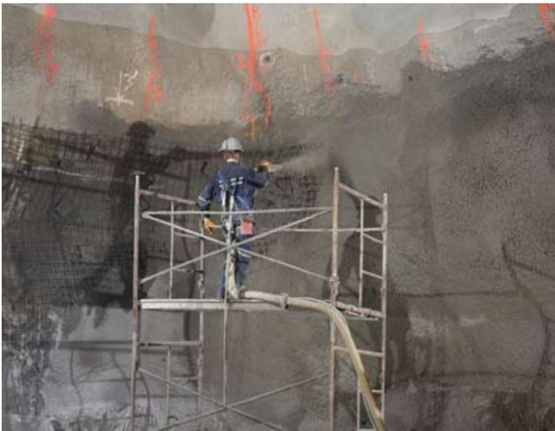
Fig. 3: Shotcreting of drift walls in progress
