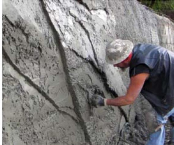
Fig. 2: Finisher carves initial fracture lines into freshly placed shotcrete
