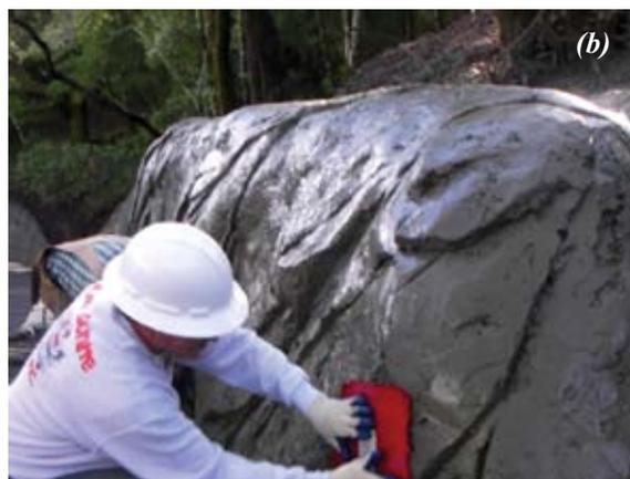
Fig. 3: (a) Texture pads; or (b) common paint rollers covered in aluminum foil impart intricate surface textures
