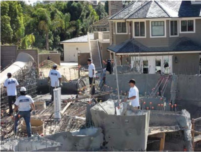
*Fig. 4: Reinforcing bar and structural shotcrete being installed in preparation for the hanging of castings*
