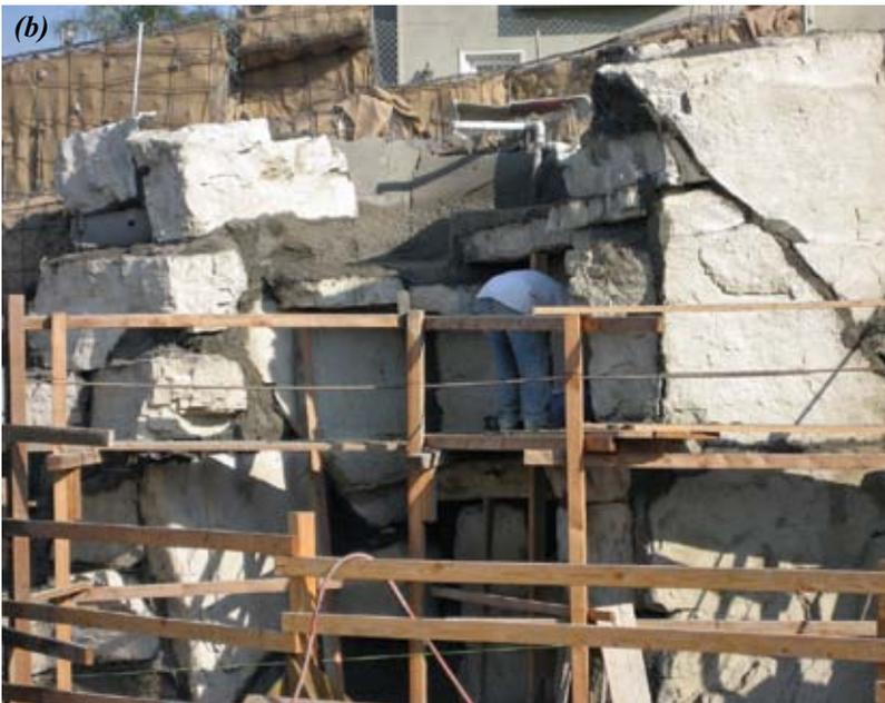
the casting panels. The rods (stainless steel) receive a nut and washer and are tightened against each of the casting panels. Once all the casting panels are installed, grout is pumped behind the casting panels, filling in all voids between the panel and the shotcrete substrate (Fig. 5(a), (b), and (c)).
