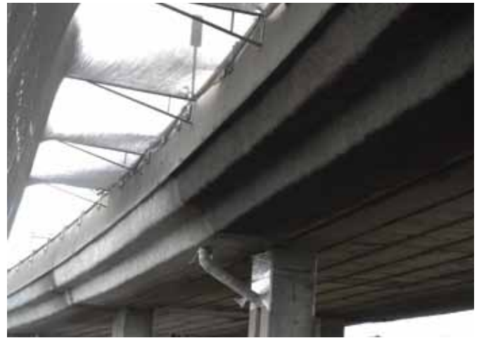
Fig. 3: Some repairs went up to 12 in. (300 mm) in thickness
