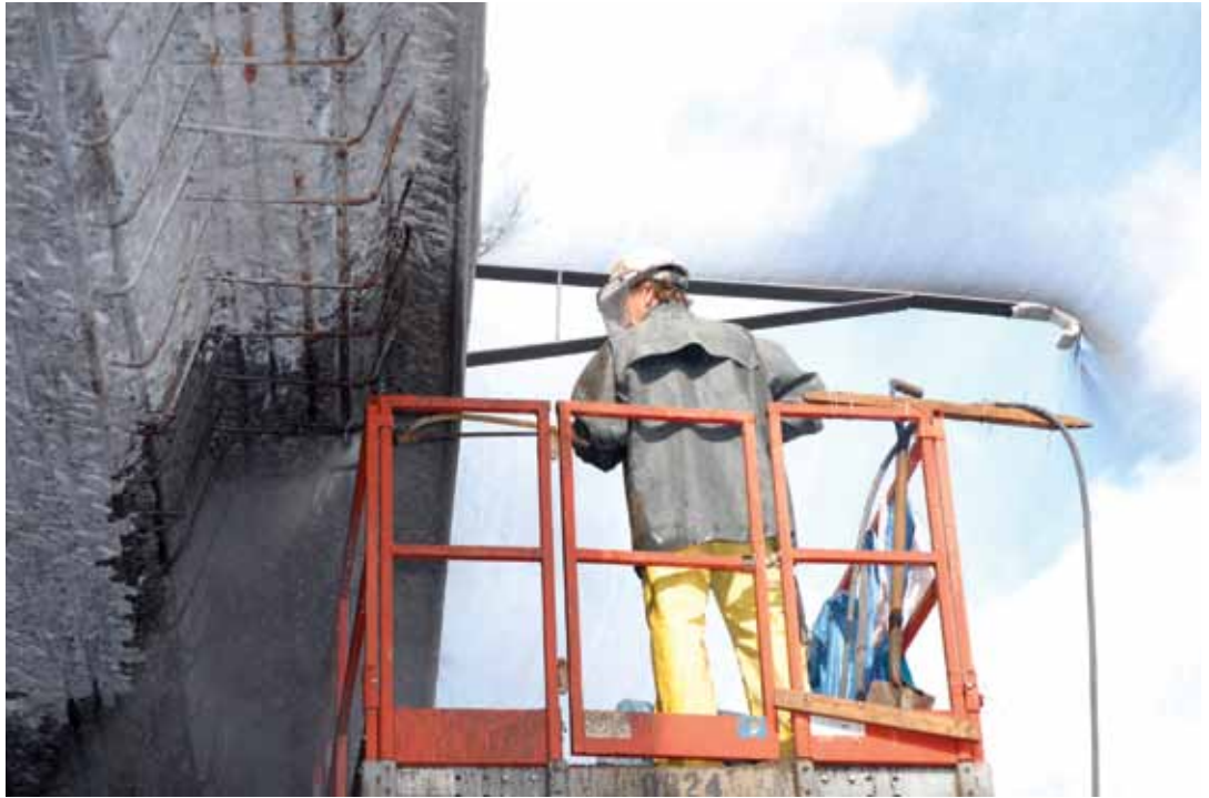
Fig. 6: The nozzleman is battling the “wind-tunnel effect”
