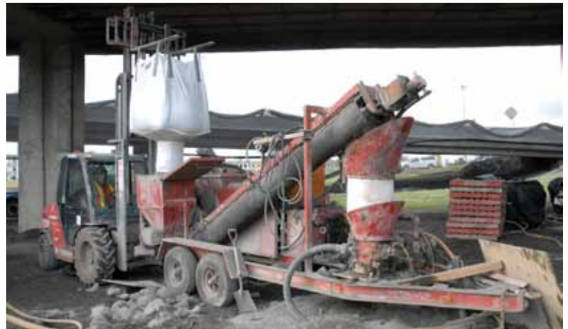
Fig. 4: With more mobile equipment, the dry-mix shotcrete process was preferred
