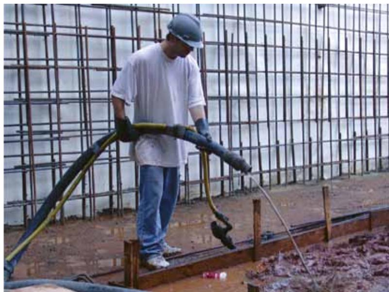
Fig 2: Line lubricant discarded outside the work area
