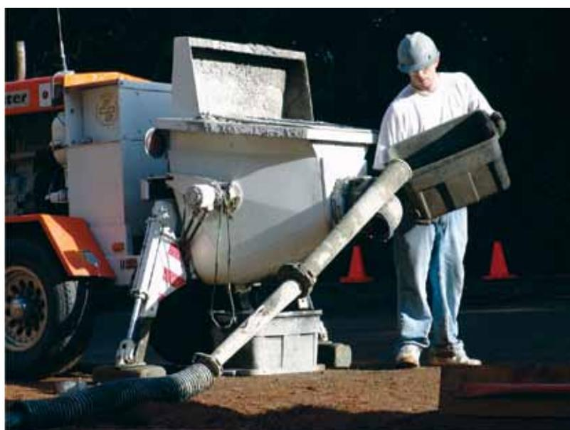
Fig 1: Line lubricant added directly to placement system
