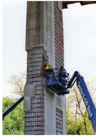
Use of the shotcrete process on the Abraham Memorial Bridge in LaSalle, IL. The contractors chose the shotcrete process following the IDOT "Structural Repair of Concrete" specification
