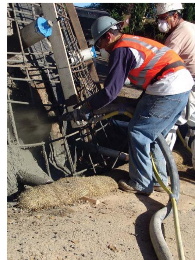
hose up, but is actually pulling downward to both bend the hose and counteract nozzle thrust. This position effectively transfers much of the placement system's weight and thrust to the ground rather than through the nozzleman's body, considerably minimizing required effort. This posture is the foundation of all effective shooting positions.
