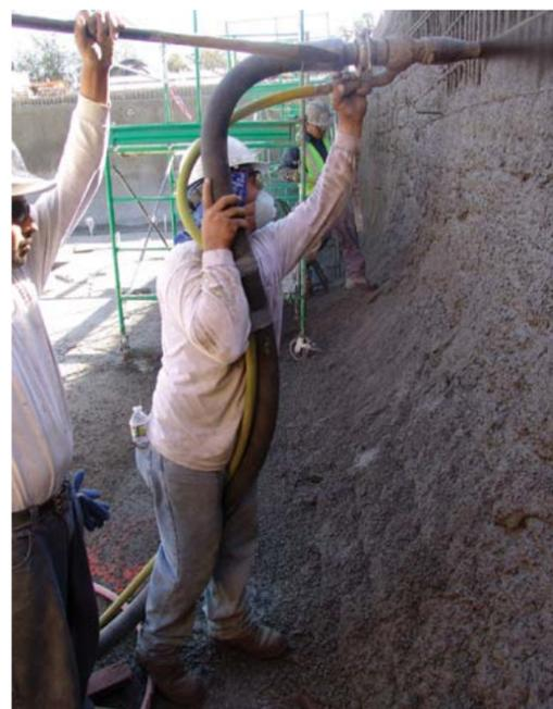
Fig. 5: Professional nozzleman works in a relaxed, well-balanced position. Note: Hose is relatively rigid and remains firmly on the ground behind the nozzleman
