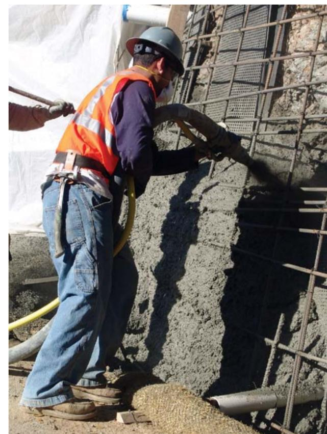
Fig. 6: Expert nozzleman maintains optimum nozzle position at various heights
