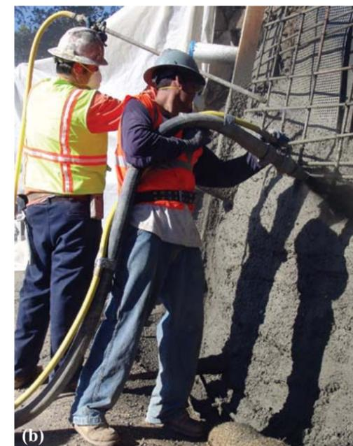
Fig. 3: Examples of awkward nozzle positions. Nozzles held (a) over the shoulder or (b) from the side reduce mobility, range of motion, and overall placement precision
