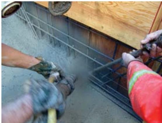
*Fig. 5: A nozzleman following a blow pipe operator and using proper techniques at the construction joint*
