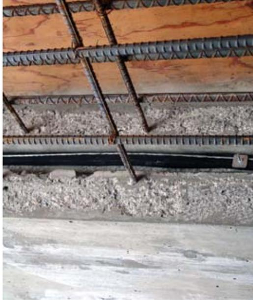
*Fig. 7: Properly installed water-stop products are important components to wall construction designs*
