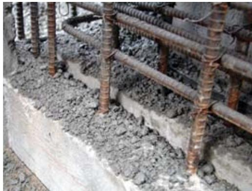
*Fig. 2: Loose aggregates collect along the construction joint ahead of the nozzle flow*
