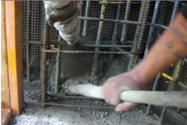
*Fig. 4: A blow pipe operator continuously removes rebound as a nozzleman places material at the construction joint*
