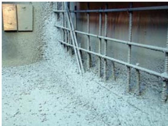
*Fig. 6: Build corners higher than adjacent areas to minimize trapped rebound*
