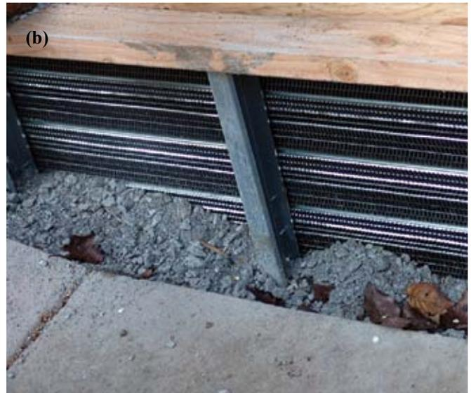
*Fig. 5(a) and (b): Completed wall after backfilling with drainage material*
