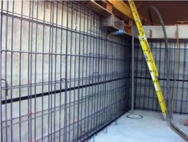
*Fig. 3: Nine-foot (2.7 m) tall wall constructed near excavated earth bank. Note drainage and waterproofing membranes applied to face side of form*
