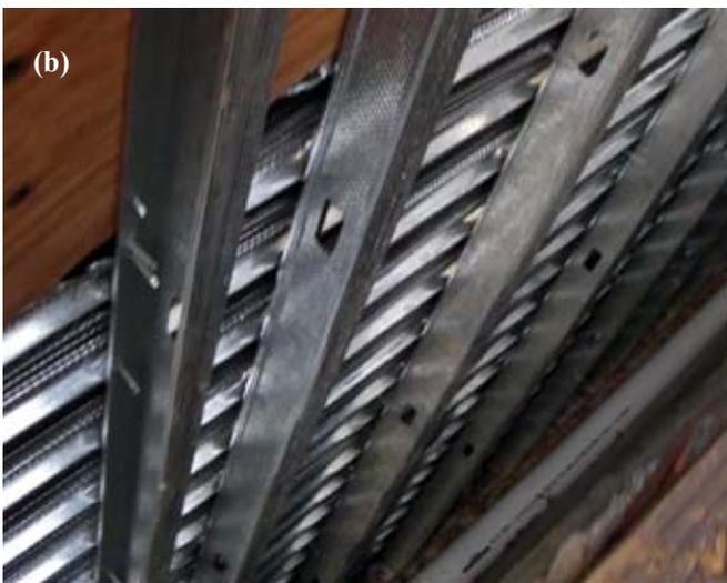
*Fig. 4(a) and (b): Back side view reveals minimal over-excavation. Alternative form materials will remain in place*
