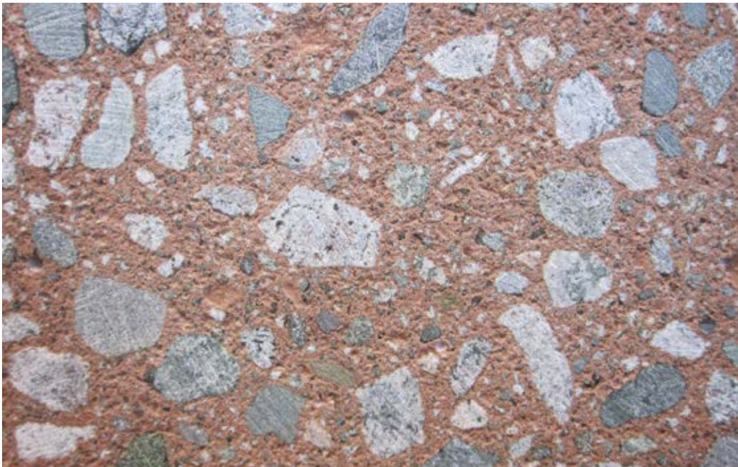
Fig. 5: Rapid-strength-gain dry-mix shotcrete modified with red pigment
