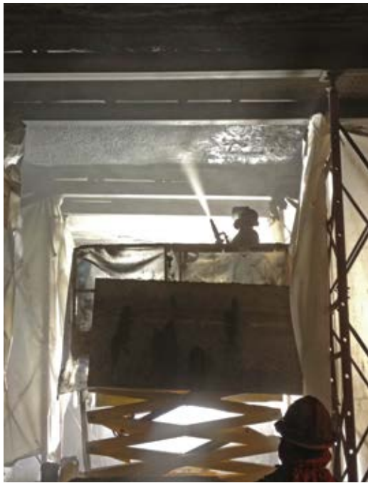
Fig. 3: Nozzlemaster shooting on the scissor lift between the temporary shoring
