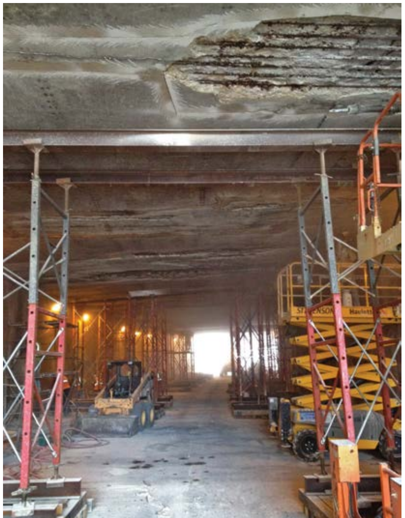
Fig. 2: Viaduct center left open for construction traffic
