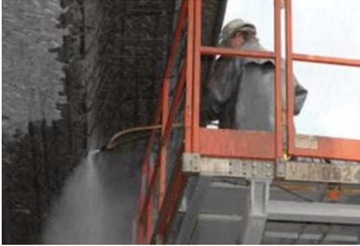
*Fig. 2: High-pressure water blasting the concrete substrate after concrete removal with a jackhammer*
