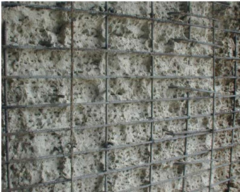
Fig. 1: A concrete surface after hydrodemolition
