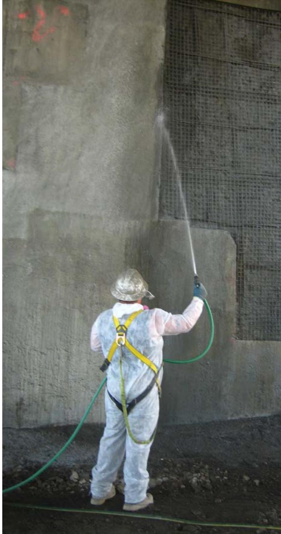
*Fig. 3: A worker prewetting the concrete substrate*
