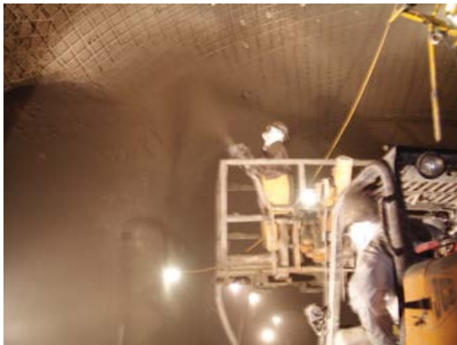
Fig. 1: Noisy job-site conditions can sometimes reduce effective communication
