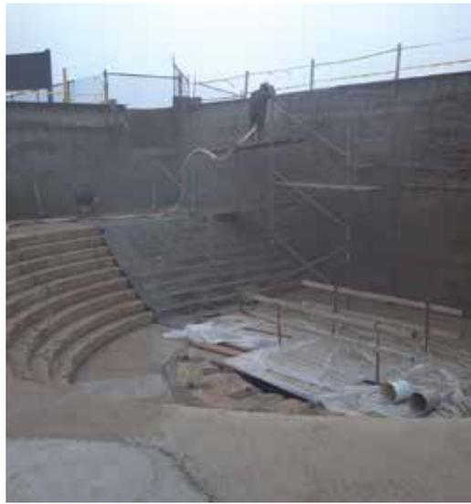
*Fig. 5: Nozzleman placing shotcrete in the cannon pit*
