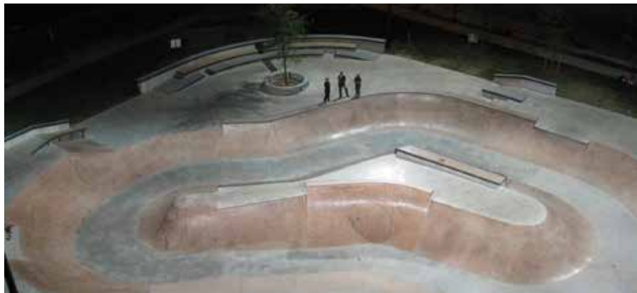
Fig. 5: North Burlington Skatepark completed
