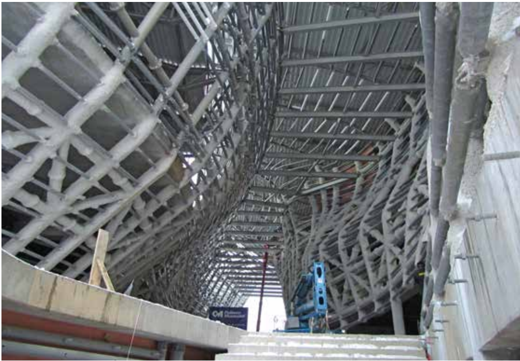
Fig. 3: Fire protected wall substructure
