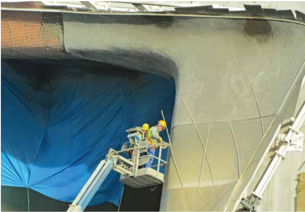
Fig. 5: Mounting of strips—control joints
