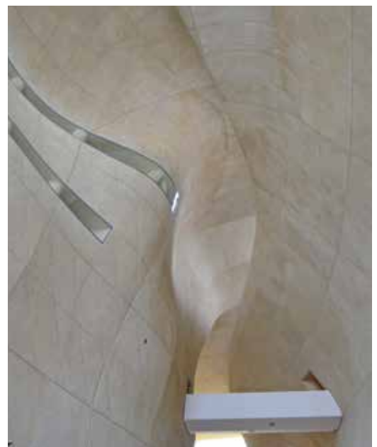
Fig. 2: "Dammed waves" of the walls in the lobby-hall area
