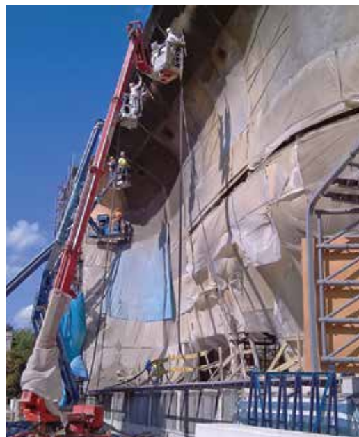
Fig. 6: Execution of top part of the wall
