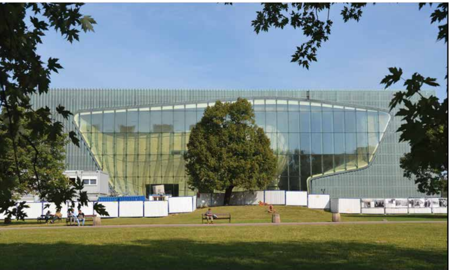
Fig. 8: A curvilinear wall with glazing (western exposure)
