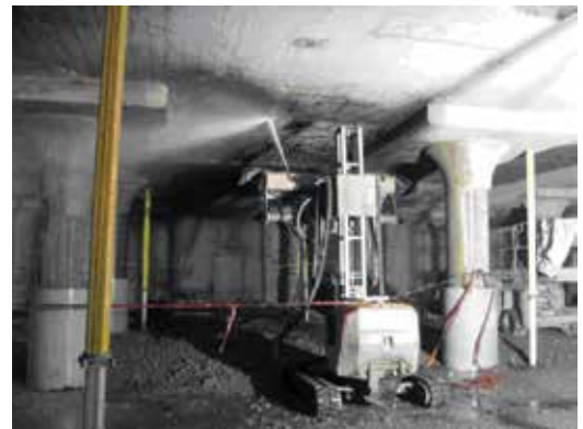
Fig. 2: The majority of concrete removals were performed by hydrodemolition
