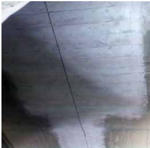
Fig. 7: New shotcrete surface to resemble 1932-formed rough-cut plank finish
