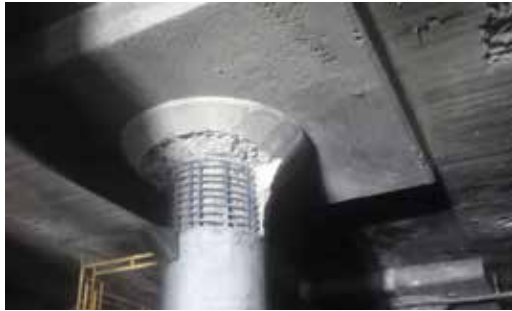
Fig. 6: Multiple layers of shotcrete prior to finish coat
