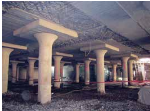
Fig. 4: Final stage of removals prior to shotcrete application
