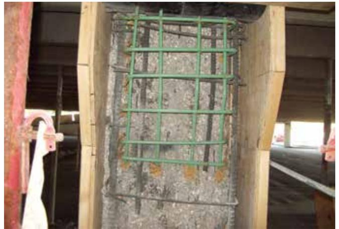
*Fig. 2: The bond characteristic of shotcrete is an important issue for the engineer because it strongly affects repair durability*
