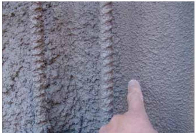
*Fig. 3: Note fine materials developing a paste layer at leading edge of the nozzle spray pattern. Although larger particles have impacted this area, they cannot embed until a sufficiently thick paste layer develops*
