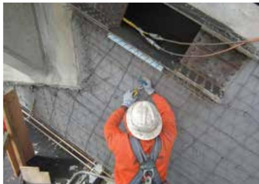
*Fig. 4: Repairing mesh prior to shoot*
