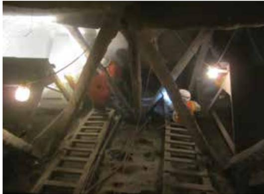
*Fig. 2 and 3: Shotcrete placement inside the arches*
