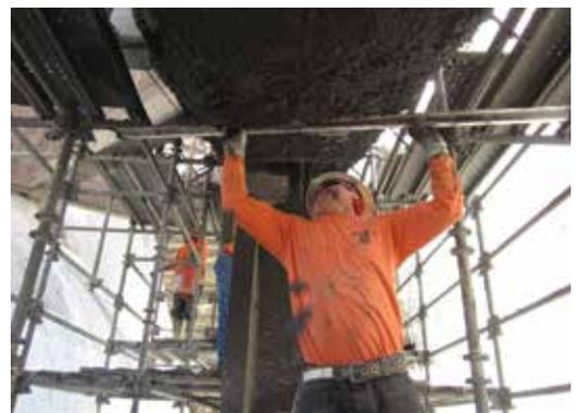
Fig. 8: Overhead finishing
