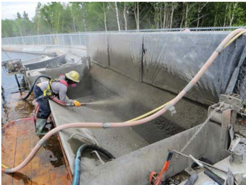
Fig. 6: Nozzleman shooting in mobile cofferdam system
