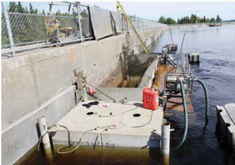
Fig. 5: Mobile cofferdam set up
