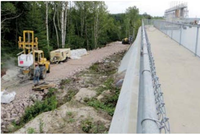
Fig. 7: Shotcrete equipment setup
