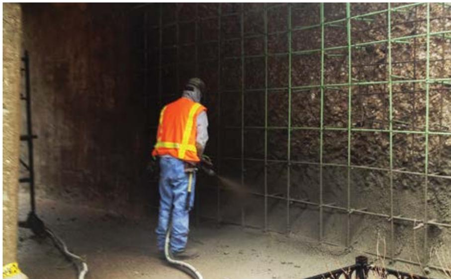
*Fig. 3: ACI Certified Nozzleman shotcreting newly-reinforced repair areas*
