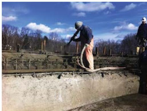
Fig. 6: Wall shotcrete and gutter detail
