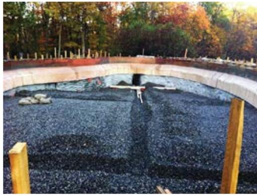
Fig. 3: Plumbing system under shotcrete shell
