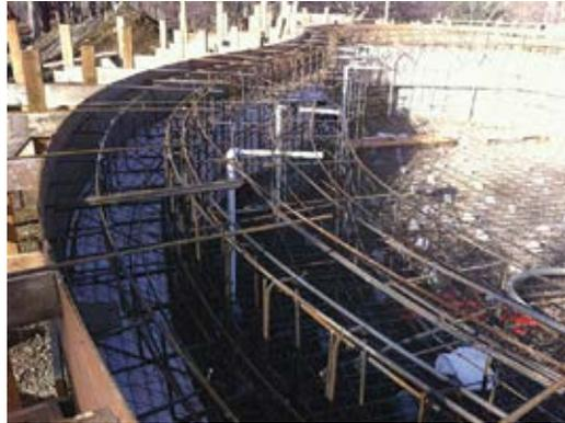
Fig. 4: Steel reinforcement on radius steps
