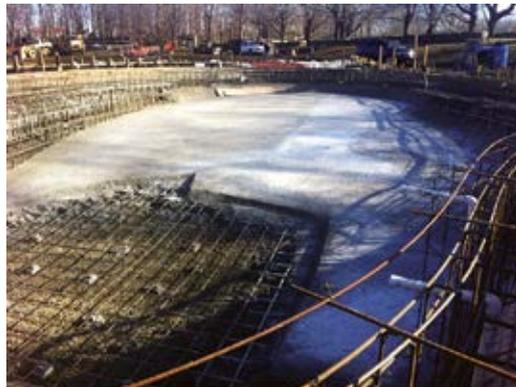
Fig. 5: Floor shotcrete (placed in stages)
