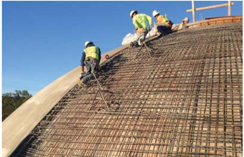
Fig. 3: Large dome shotcrete preparation
