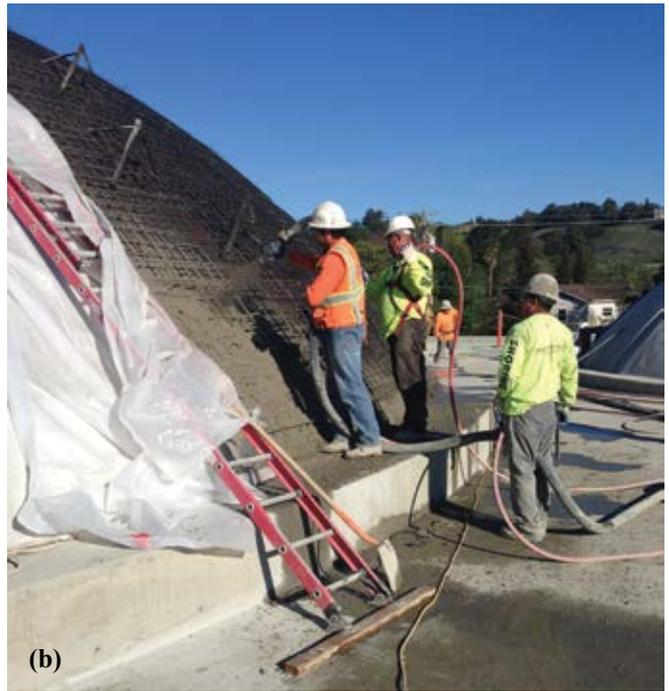
Fig. 2(a) and (b): Large dome shotcrete installation
