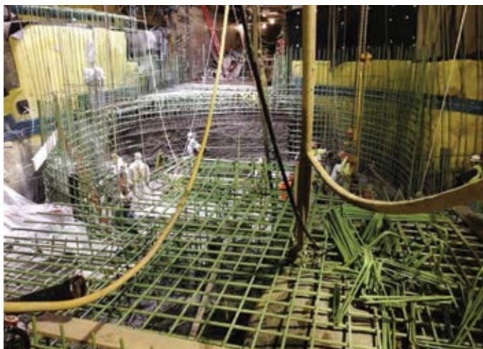
Fig. 1: Shaft structure—shot two water barrier panels per shift
