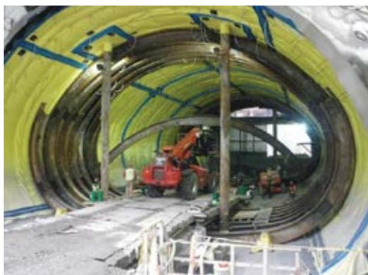
Fig. 4: Waterproofing and ring girders being installed
