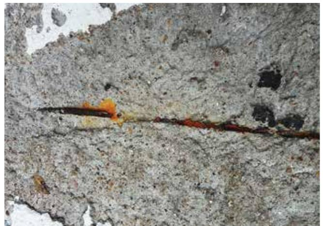
Fig. 6: Insufficient coverage over reinforcement. Reinforcement bowed outward
