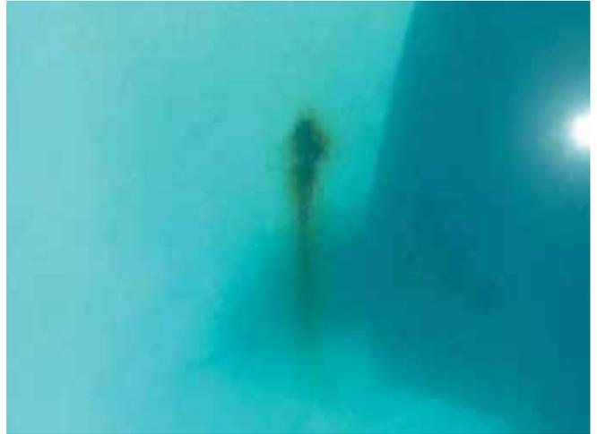
Fig. 8: Rust bleeding through a plaster finish of a swimming pool due to reinforcement corrosion
