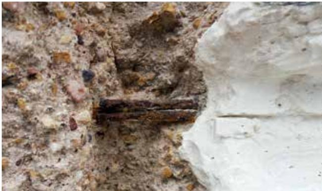
Fig. 4: Macro void space (air pocket) around reinforcement and bar termination bent upward
