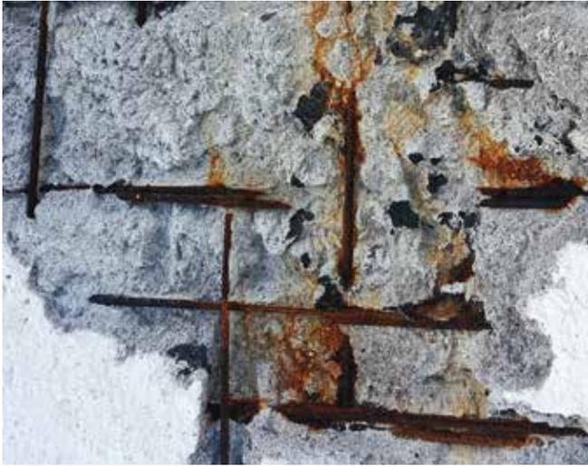
Fig. 7: Complete corrosion of reinforcement grid due to inadequate coverage. Corrosion reaction creates internal stress and delamination of cover material
