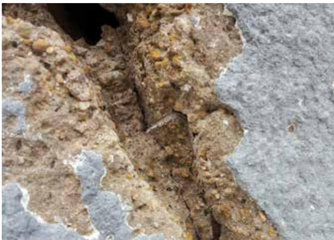
Fig. 5: Structural crack created pathway allowing chemical bridge to initiate corrosion
