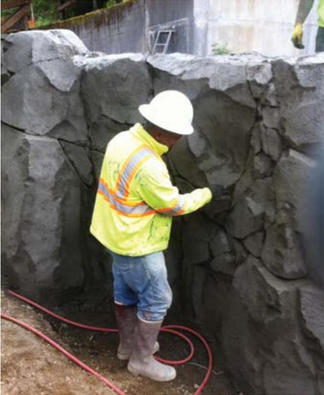
Fig. 4: Shotcrete finishing for bedrock textures
