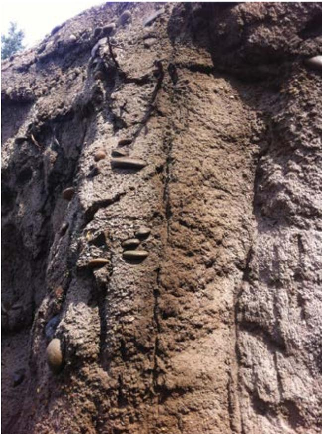
Fig. 2: Earthen textures with embedded cobbles, roots, integral pigments, and topical stains
