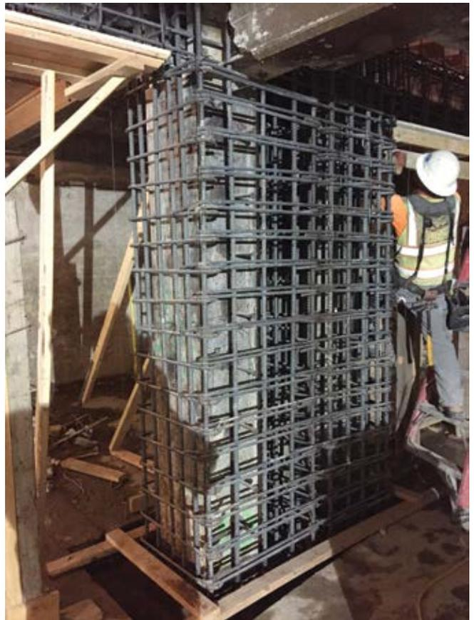
Fig. 2: Column encasement and shear walls reinforcement on the first-floor level
