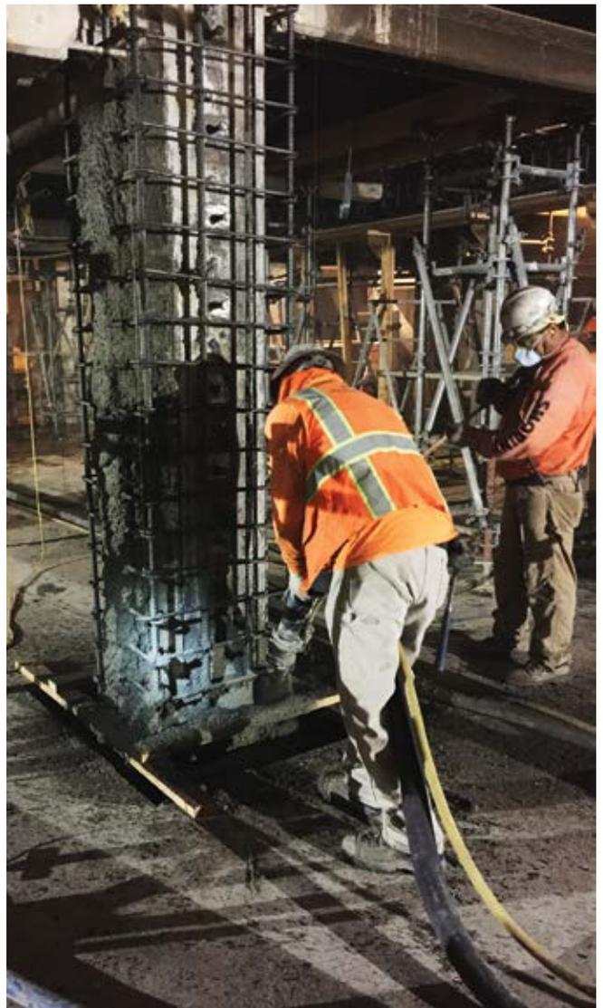
Fig. 4: Shotcrete installation for column encasement
