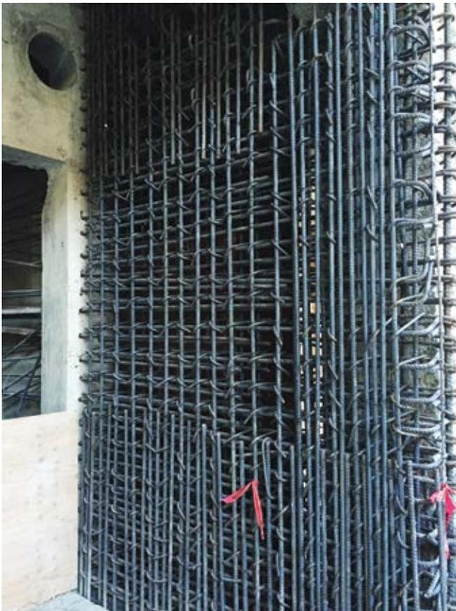
Fig. 1: Typical reinforcement for shear walls and boundary elements on the fourth floor
