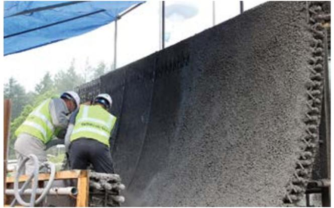
Fig. 5: Shotcreting the sliding track wall
