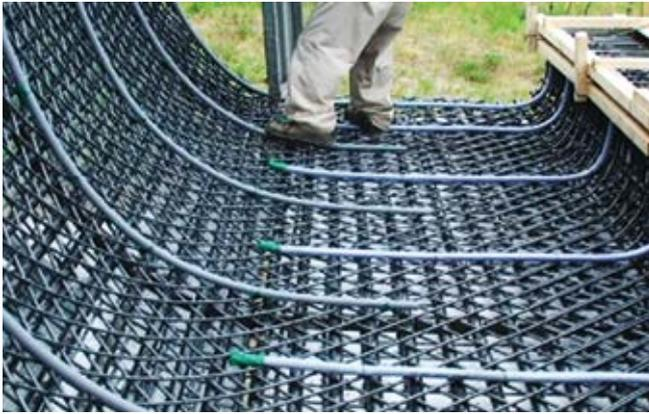
Fig. 4: Track section ready for shotcreting
