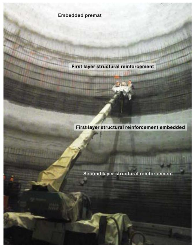
Fig. 9: View showing multiple phases of dome building process. Domtec shotcrete technicians average over 25 years of experience each
