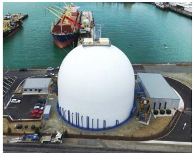
Fig. 2: Aerial view of Holcim Cement Terminal in Timaru, New Zealand. Dome is 118.1 ft (36 m) in diameter and 103.3 ft (31.5 m) tall and stores 33,000 tons (30,000 tonnes) of cement powder and used 1923 yd<sup>3</sup> (1470 m<sup>3</sup>) of shotcrete to construct
