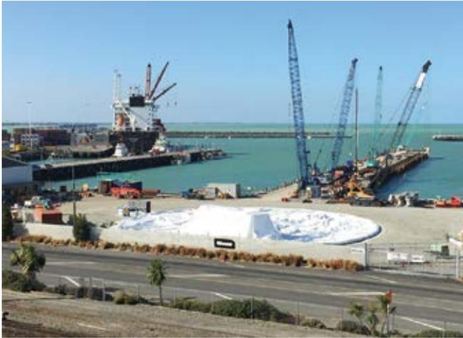
Fig. 6: Timaru dome air form ready for inflation. The DomeSkin™ air form is 38,350 ft<sup>2</sup> (3563 m<sup>2</sup>)
