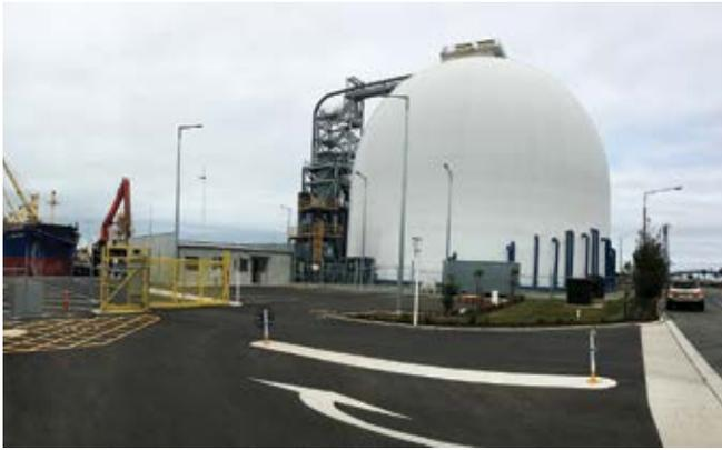
Fig. 3: Street view of Timaru cement storage dome. Aesthetics were a major consideration when deciding on a storage solution. The dome durability, white fabric color, insulation, price, and Domtec's reputation also figured into the contract award
