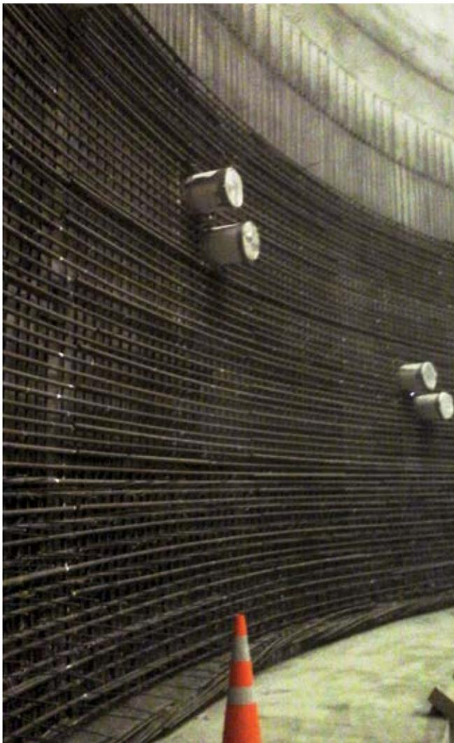
Fig. 8: Typical dome structural reinforcing bar mat; over 550 tons (500 tonnes) of reinforcing bar was used in the Timaru dome
