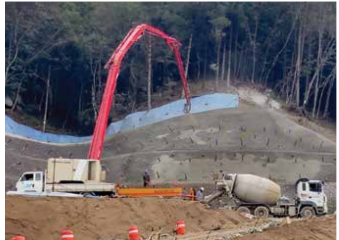
Fig. 3: Construction of tunnel portal using cellular sprayed concrete
