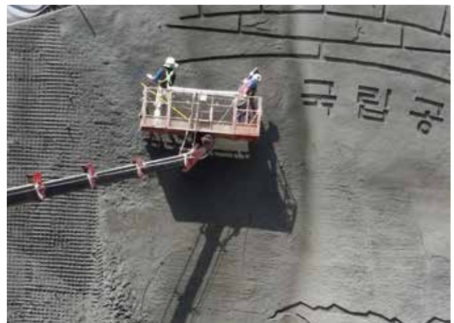
Fig. 4: Spraying at tunnel portal
