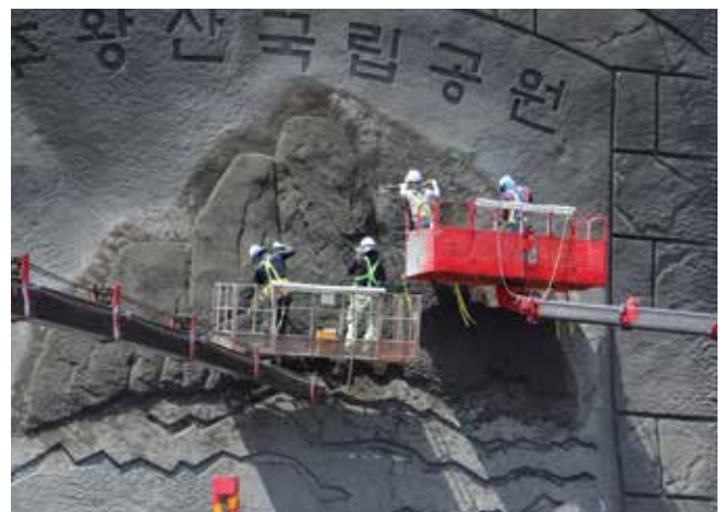
Fig. 5: Carving regional symbol at tunnel portal
