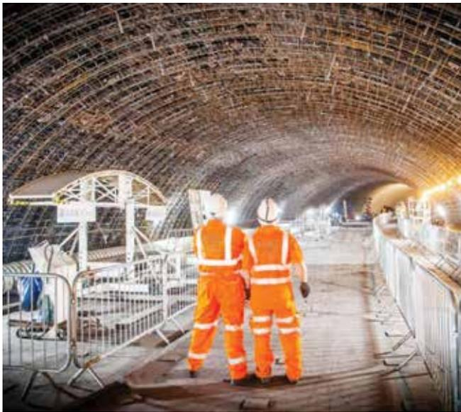
Fig. 5: 990 RAM Arch reinforcement units installed. Bespoke arch lifting machine shown to the left
