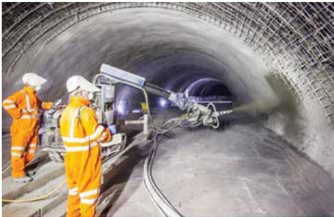
Fig. 7: Robot sprayer at work. Remember there are trains running beneath this!
