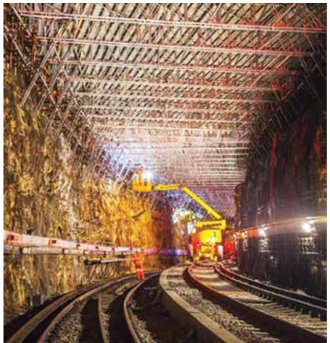
Fig. 3: The access deck from track level
