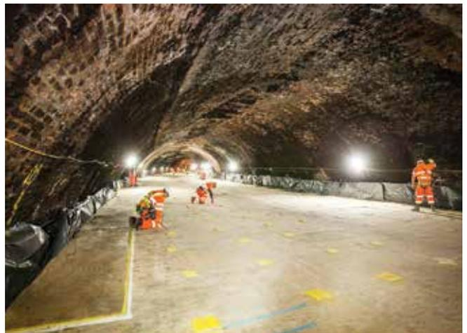
Fig. 4: A fully segregated working platform is created with trains running below
