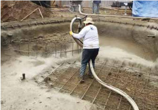
*Fig. 5: SSG used dry-mix shotcrete for this smaller pool with about 50 yd<sup>3</sup> (38 m<sup>3</sup>) of concrete and easily completed in 1 day with dry mix. Additionally, the steel schedule was light and with a tight jobsite it is easier to clean up a dry-mix setup than a wet-mix setup*
