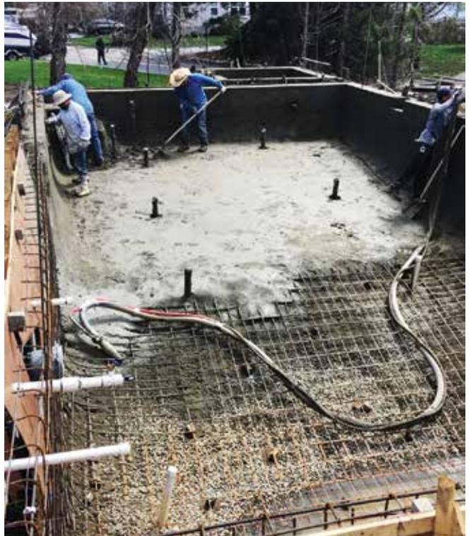
Fig. 2: The crew is able to walk on recently shot dry-mix material without sinking into the surface
