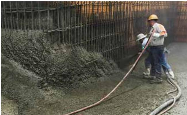
Fig. 3: Wet-mix shotcrete was used on this pool because of the congested reinforcing bar layout, as well as requiring about 300 yd<sup>3</sup> (230 m<sup>3</sup>)
