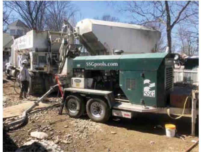
*Fig. 6: Wet-mix shotcrete pump and on-site volumetric mixer allowed for faster production, as there was no swapping out of concrete trucks*
