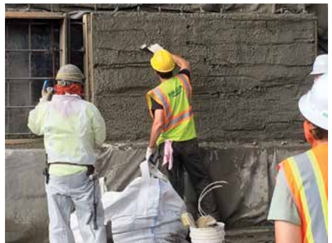
Fig. 3: Mockup immediately after spraying and early stages of sculpting
