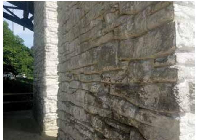
Fig. 2: Precast panel installed at the bottom of the pier
