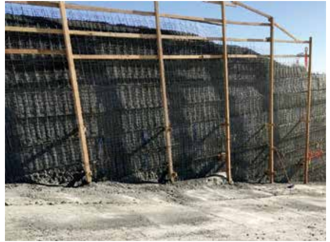
Fig. 5: Shotcrete substrate of RCC berm and WWF reinforcing
