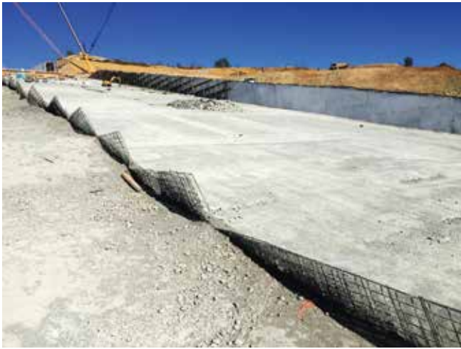
Fig. 3: RCC berm supporting main spillway walls
