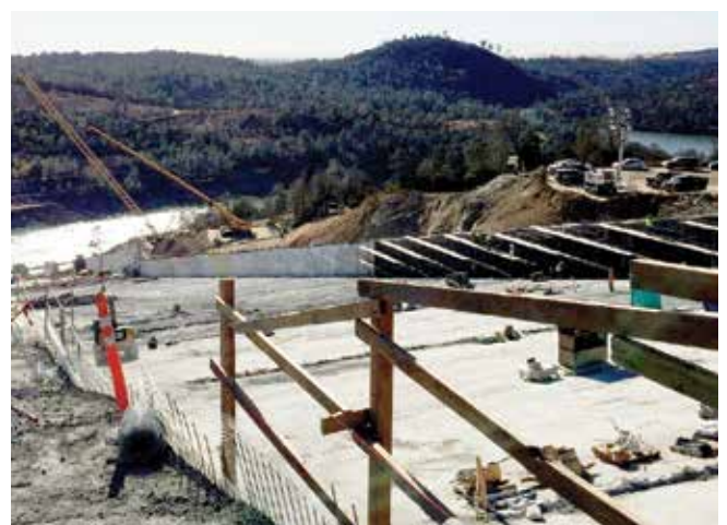
Fig. 7: View looking down spillway chute at temporary shotcrete walls
