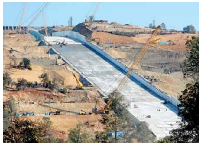
Fig. 2: Middle third of the 3000 ft (900 m) main spillway chute
