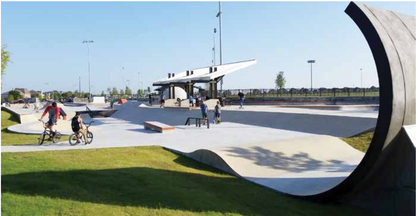
Fig. 4: Over-vertical, cantilevered concrete wave feature in foreground
