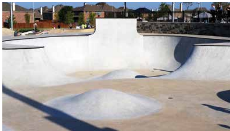
Fig. 2: Flow bowl section with speed and direction control features on the floor. A 6 ft (1.8 m) tall wall extends above the coping line
