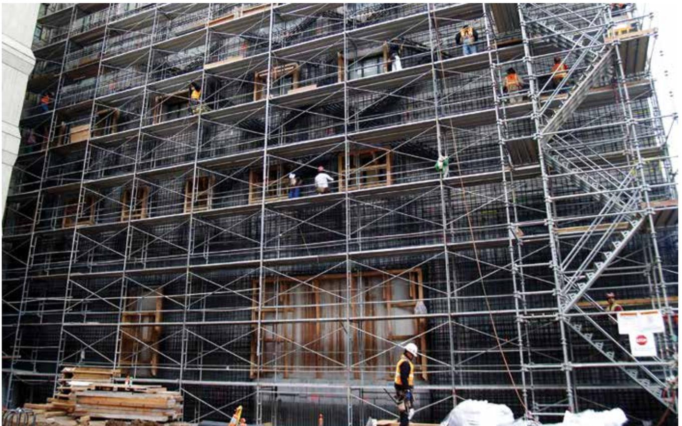
*Preparing for shotcrete placement on a building seismic retrofit*
