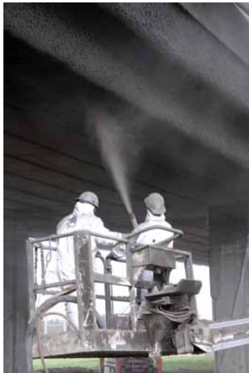
Fig. 7: A repair zone is blasted to clean the reinforcing bar and the substrate
