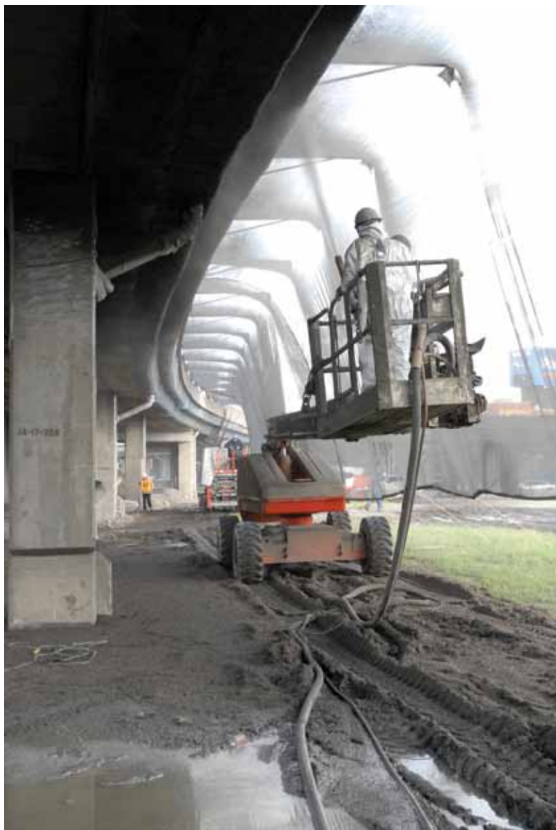
Fig. 9: Applying shotcrete from a distance of 2 to 6 ft (0.6 to 1.8 m)
