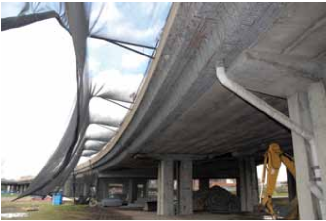
Fig. 2: More than 4600 linear ft (1400 linear m) of repairs were required
