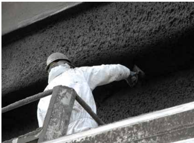
Fig. 10: The rough finish was achieved with a steel trowel
