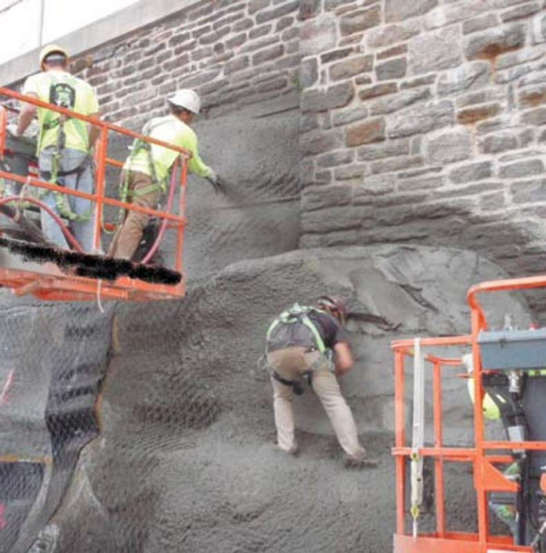
Fig. 4: Applying and sculpting shotcrete
