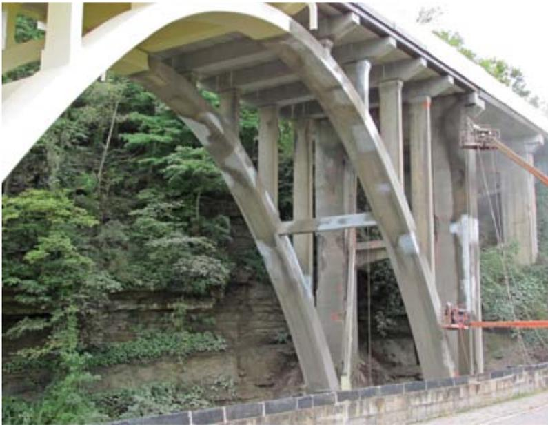
Fig. 4: Open spandrel arch and spandrel column rehabilitation
