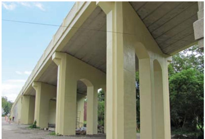
*Fig. 3: Rehabilitated columns with tintable epoxy urethane sealer*
