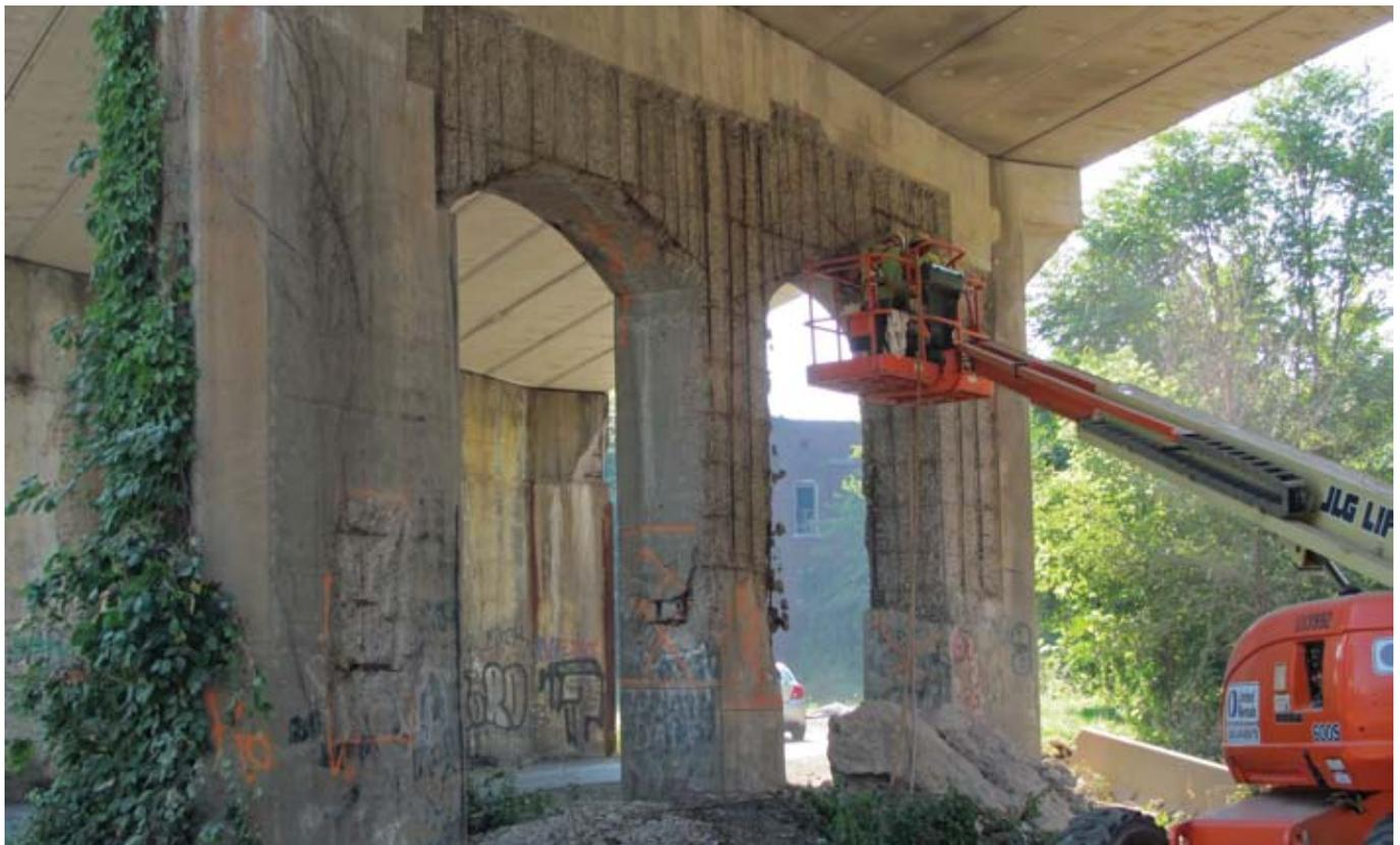
Fig. 1: Deteriorated concrete being removed during demolition
