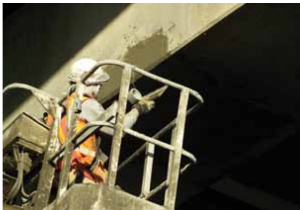
11,000 ft 3 (311.4 m 3 ) of removal and replacement
