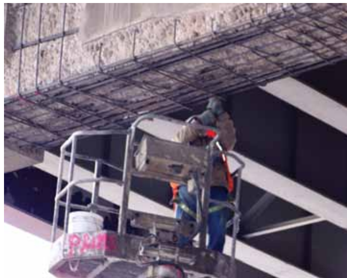
Over 15,000 lb (6803.8 kg) of reinforcement was supplemented
