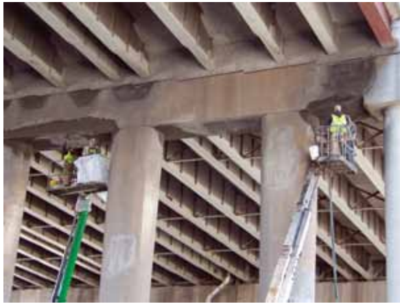
Completed by American Concrete Institute (ACI) Certified Nozzlemen
