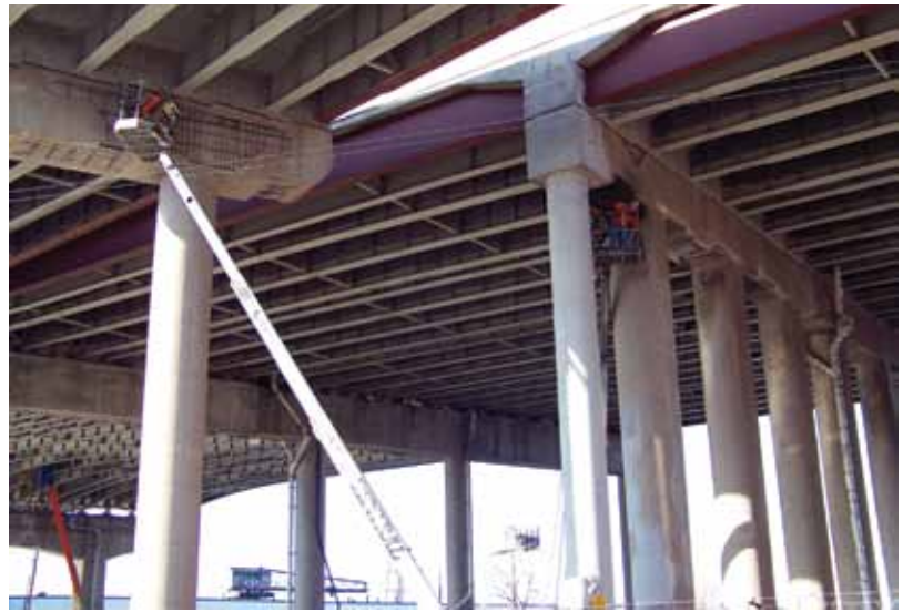
A 60 ft (18.28 m) boom lift was used to access piers
